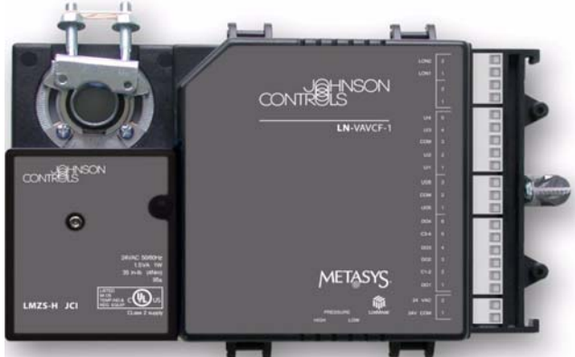
Figure 1: LN VAV Controller
